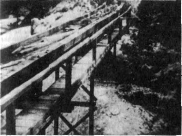
Logging Flumes in Neuburg.
